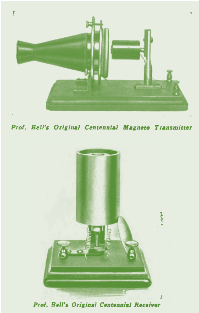
Alexander Graham Bell's transmitter and receiver for the first telephonic telegraph (1876–1877).
